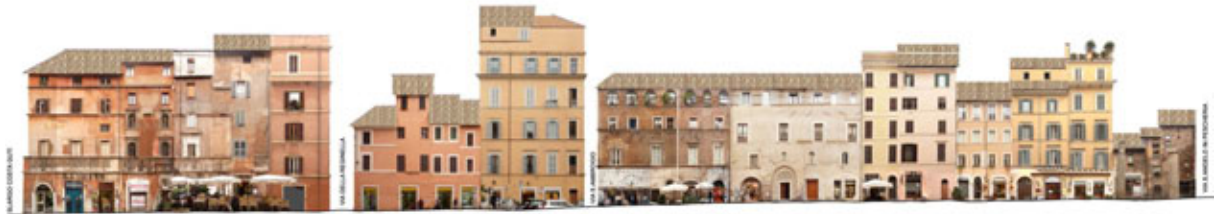
Fig. 4: Survey. Photoplan ( fotomosaicatura ) of the whole facades. Thus, it is also evident material and colorimetric aspects of the building curtain.
